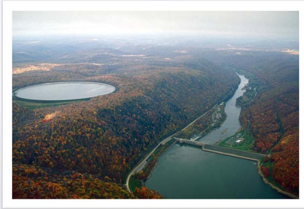
Seneca Pumped Storage Station and Kinzua Dam
