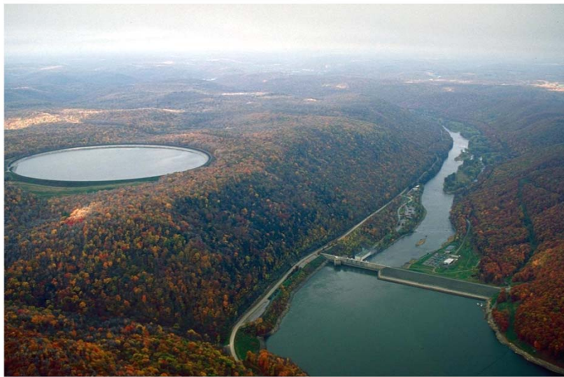
Seneca Pumped Storage Station and Kinzua Dam
